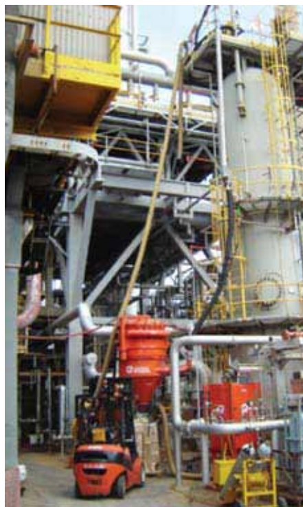
01. Vacuum unloading of Catalyst 02. Loading a basket using the Casale nozzles 03. Technicians use a CR Drum Decenter on site for the efficient loading of Hoppers and Bags 04. Vacuum unload of catalyst 05. Spent catalyst stored in UN approved containers 06. Confined Space Dense Loading in progress
